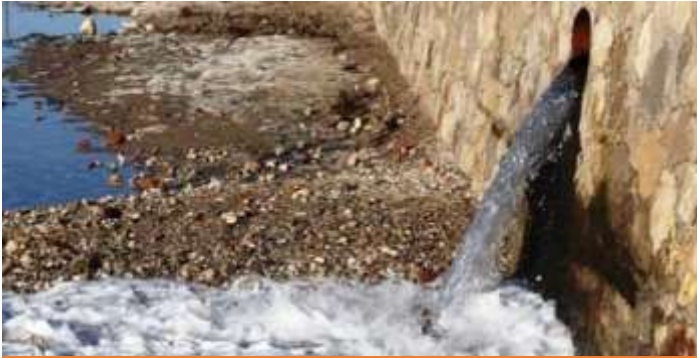
Interconnection of storm water & sewerage networks. Photo: untreated sewage discharged into Mithi
